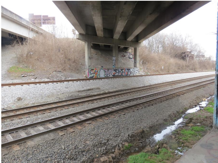
BENT #1 - BACK VIEW
