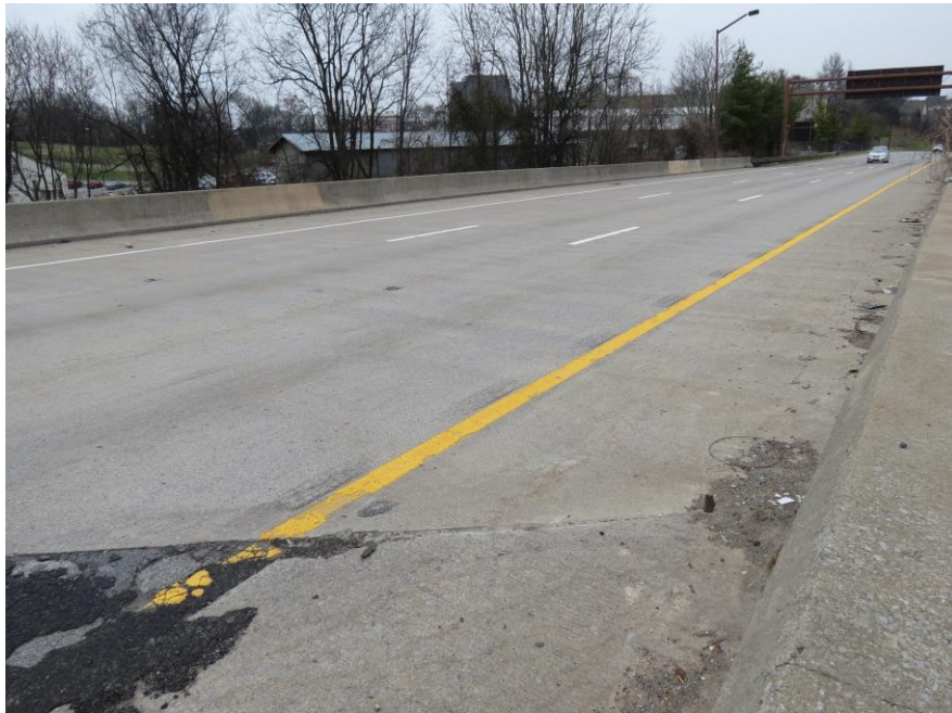
VIEW ACROSS TOP OF WEARING SURFACE
