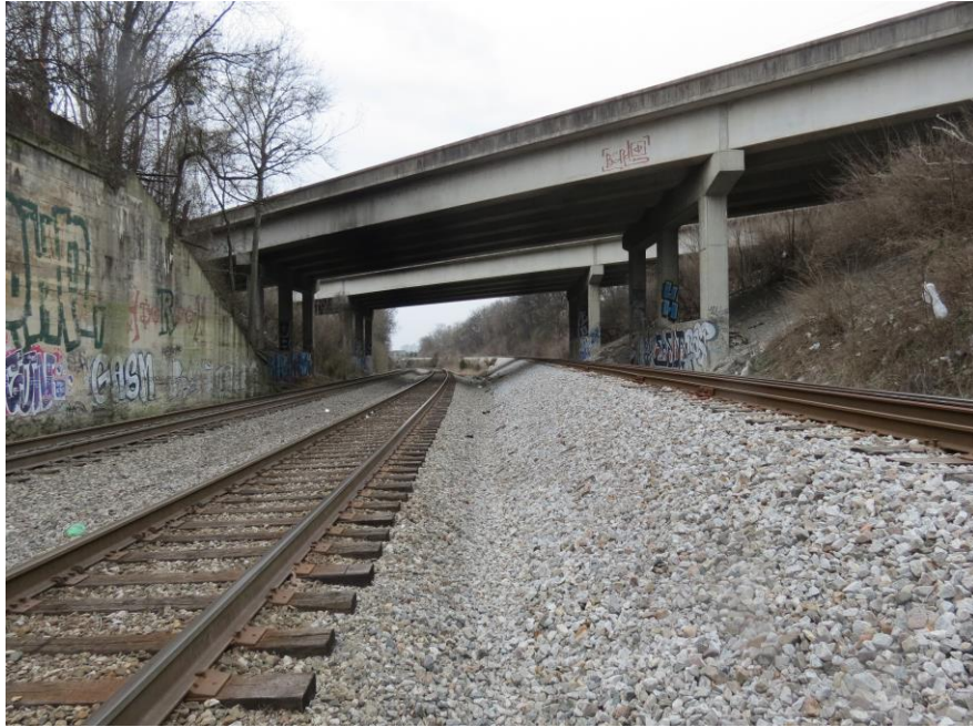
CLEARANCE VIEW LT. SIDE
